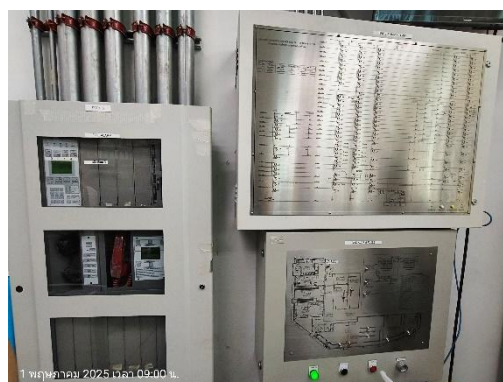
fire alarm control Panel
